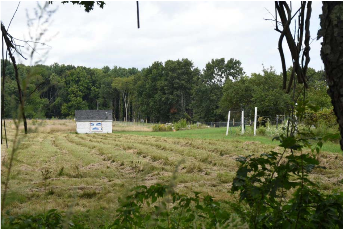
Figure 9. View of SRP transmission corridor from Little Bay Road, facing north.
